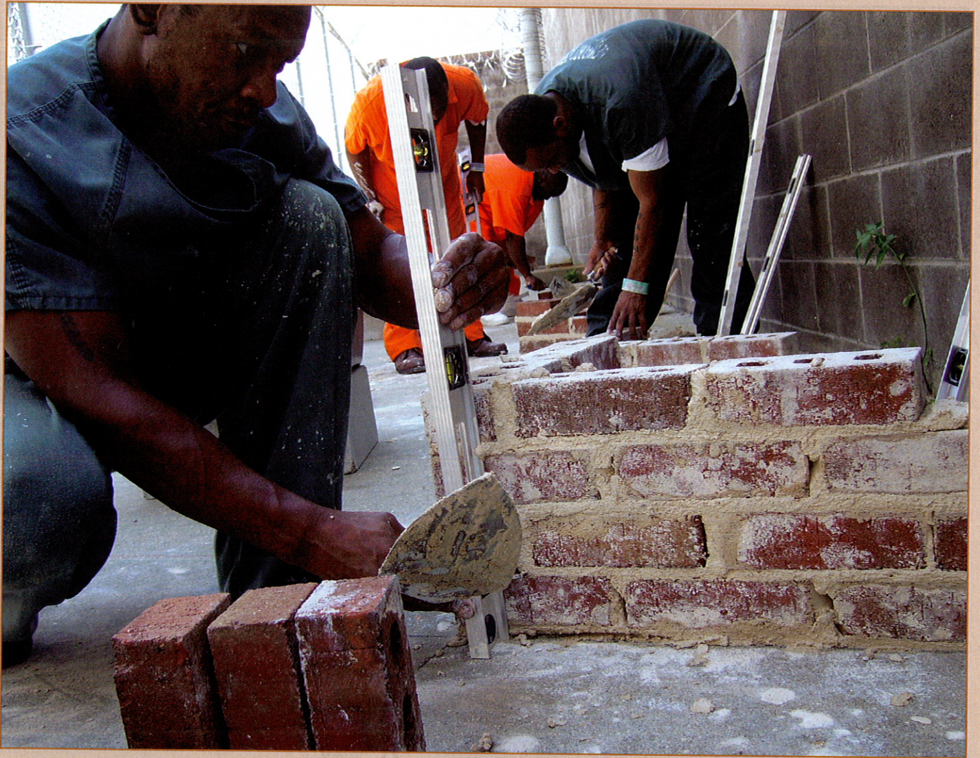
Inmate inspects wall
