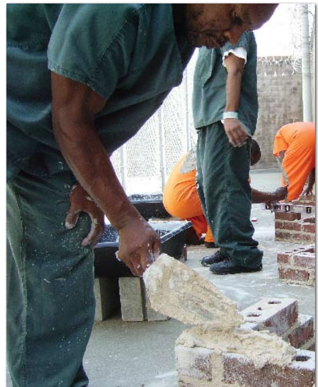
Inmates spread mortar and level walls.
